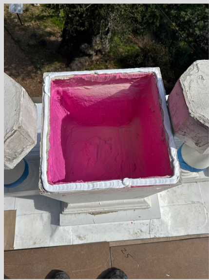
Inside the railing, sealed and fixed
