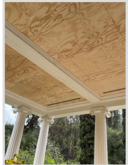
Rebuilding the frame
